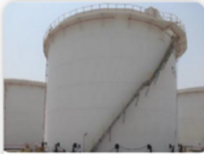
JACKING SYSTEM FOR STORAGE TANKS REPAIR
