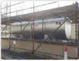
FABRICATION & INSTALLATION OF HORIZONTAL TANKS
