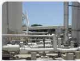
INSULATION & CLADDING WORKS
