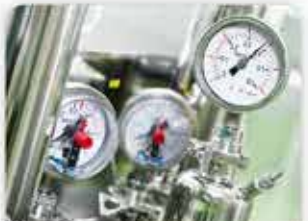
TANK HYDROSTATIC TESTING
