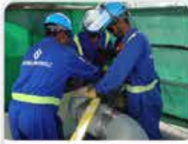
ONSITE PIPING INSTALLATION WORKS
