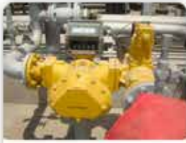
FLOW METER CALIBRATION & INSTALLATION
