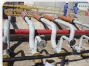
MECHANICAL SITE WORKS
