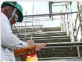
SCAFFOLDING INSTALLATION, INSPECTION & CERTIFICATION
