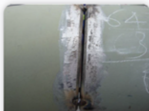
PIPING WELDING WORKS
