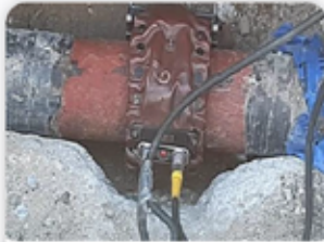
LRUT INSPECTION OF UNDERGROUND PIPELINES
