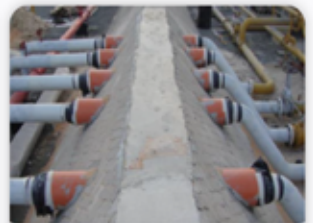
PIPING FABRICATION & INSTALLATION
