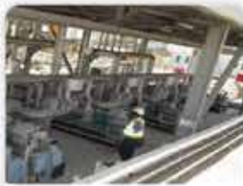
PUMP HOUSE INSPECTION
