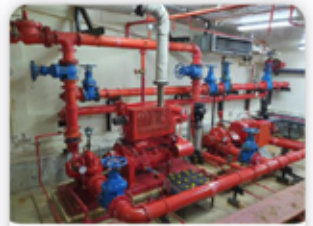
FIRE FIGHTING SYSTEM INSTALLATION & MAINTENANCE
