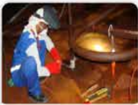
INSIDE TANK REPAIRS & MAINTENANCE
