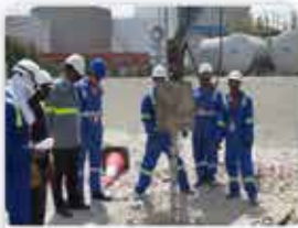
INSTALLATION OF GROUND WATER MONITORING SYSTEM
