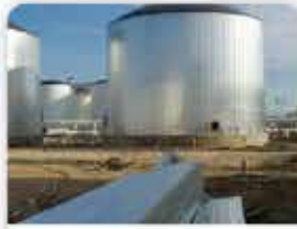
BITUMEN FACILITIES INSPECTION & ENGINEERING SUPPORT
