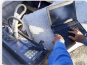
INSPECTION OF MEP EQUIPMENTS
