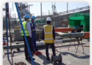
ONSITE PREFABRICATION WORKS
