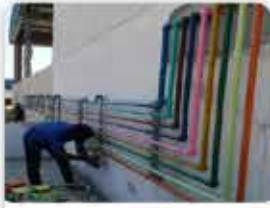
INSTALLATION OF UTILITY LINES
