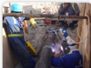
UNDERGROUND PIPELINE WORKS
