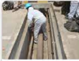
PIPELING TRENCH CONSTRUCTION
